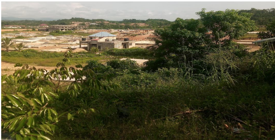
Figure 2: A picture of the town with reconstruction going on.
